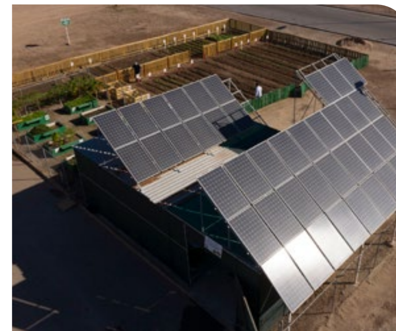
Mexicali, Mexico MODCO facility
