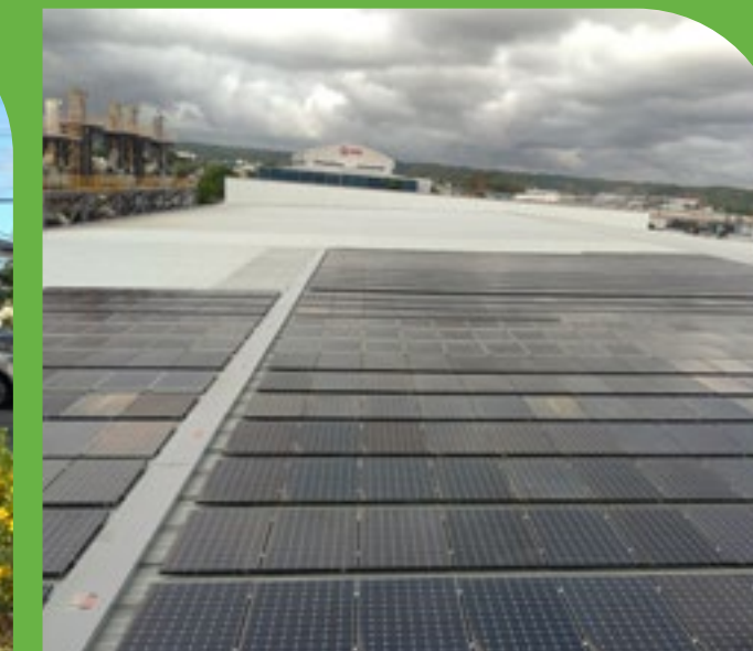
Installation of Solar Panels at the South Main Roof
