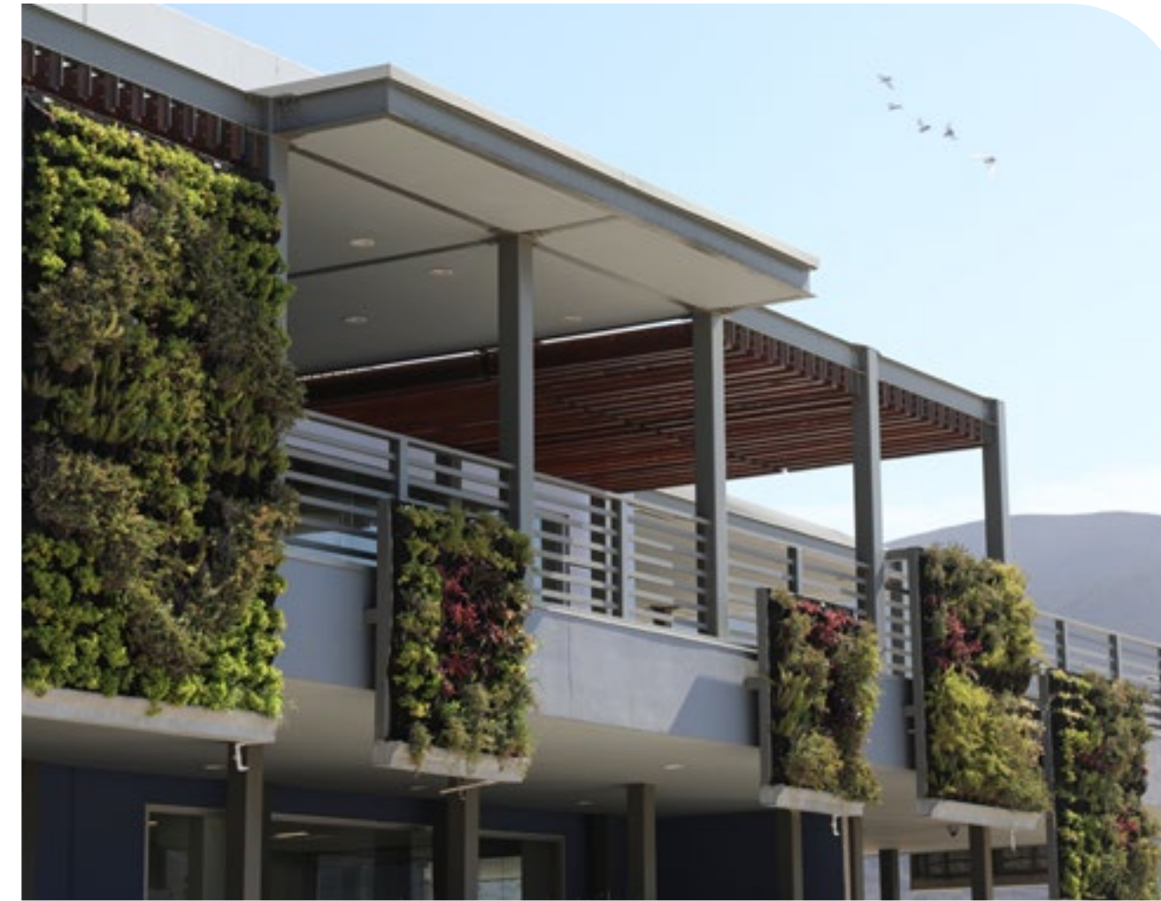
Ensenada, Mexico MODCO facility
