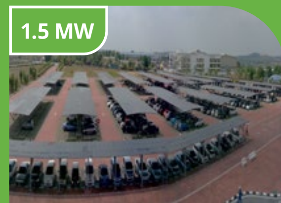
3. Covered carpark and motorcycle area
