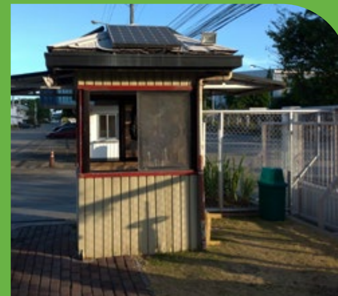
Installation of Solar Panel at the Security Post
