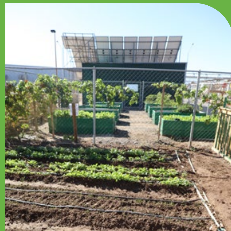
Solar panels installed atop our organic garden
