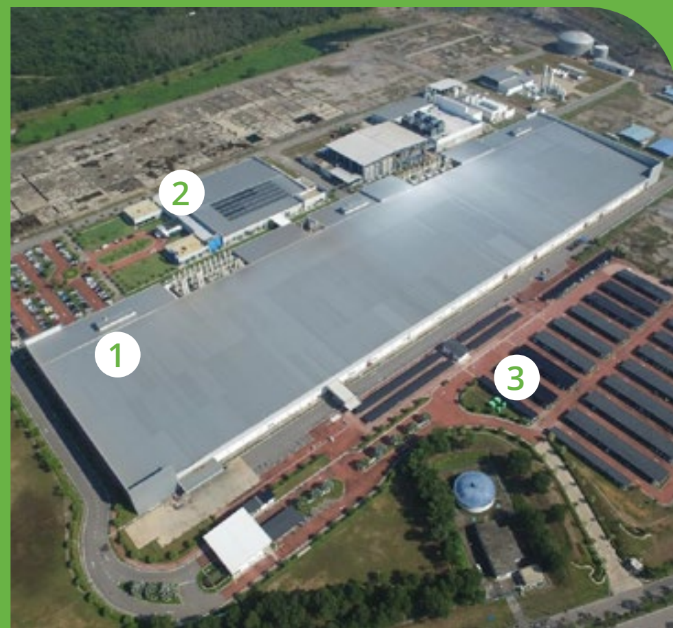
1. Future planned – FAB rooftop
